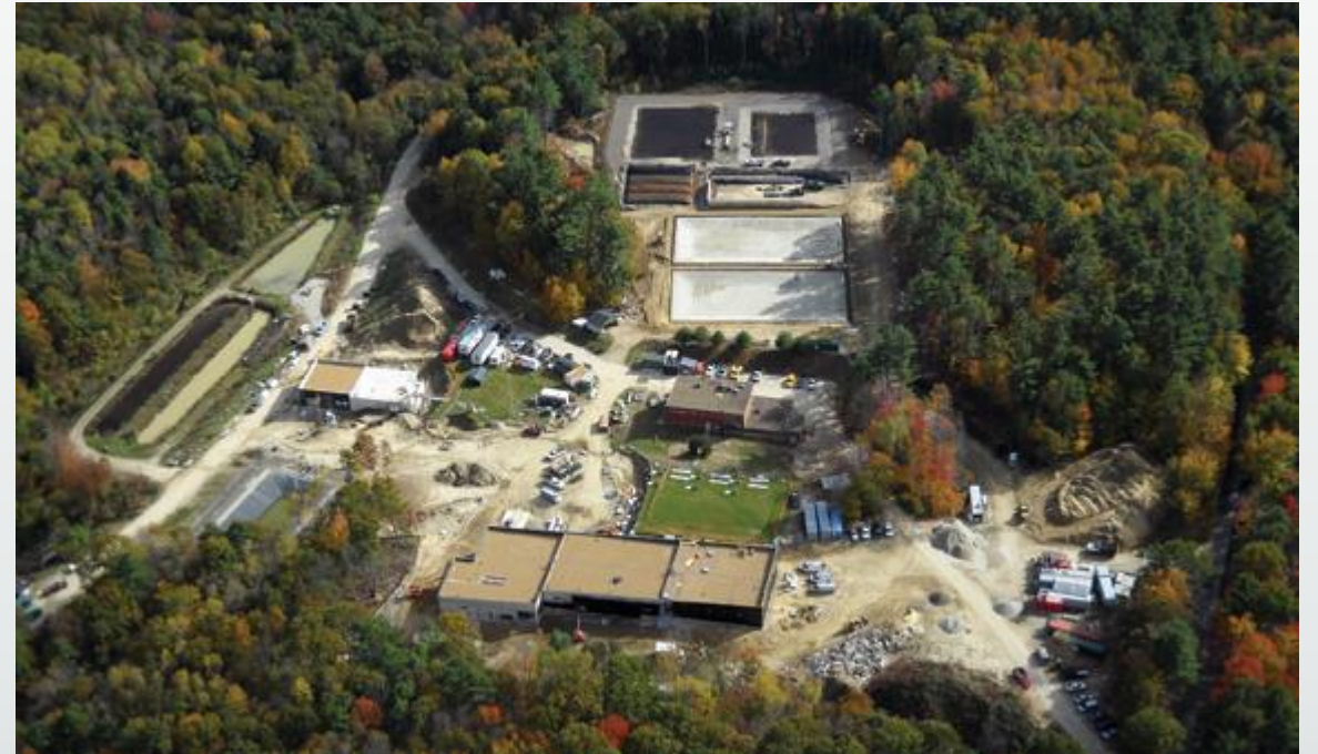
Portsmouth Water Treatment Plant
